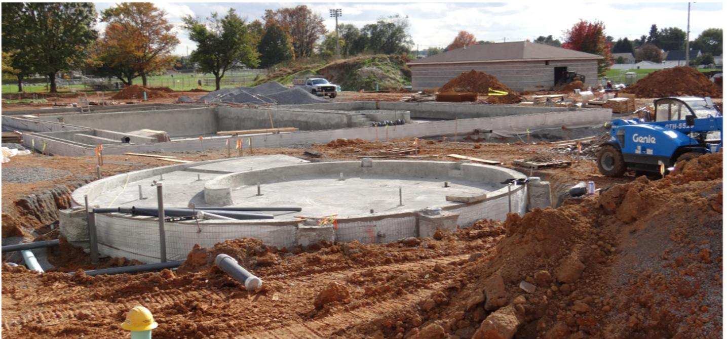
**The two pictures below depict the skeleton of the Lazy River. The exterior walls will be sprayed, and then the final shotcrete process will be applied to the walls of the center island. Upon this completion, all pools will be ready for the final, applied finish and then filled!**
