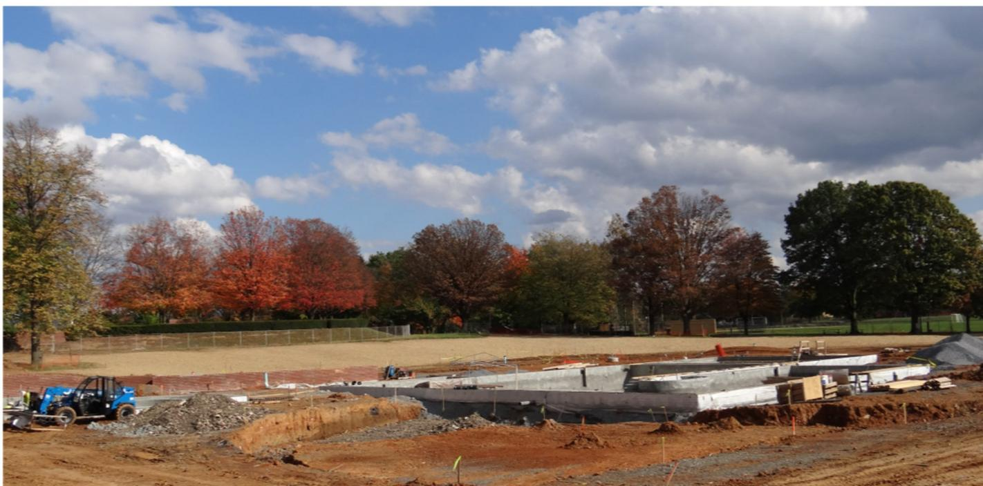
**The concrete on the upper deck has been poured, and the steps and retaining walls are in place. Decorative fencing will be installed to comply with building code requirements relative to fall heights.**
