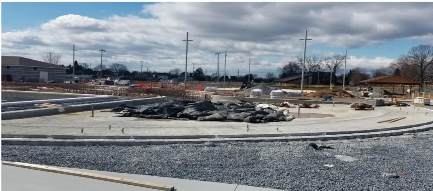
**Above: Current completion of the formation of the beach-entry of the Leisure Pool which is finished and awaiting the installation of the play structure.**
